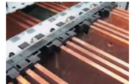
^ 1 to 3 bars, 10 mm thick, per pole
