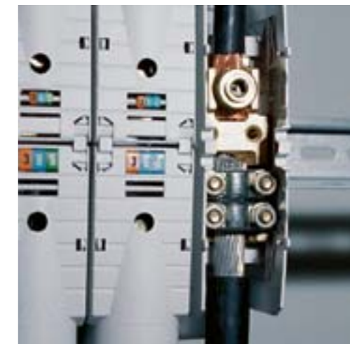
< Alumin./copper direct connection
