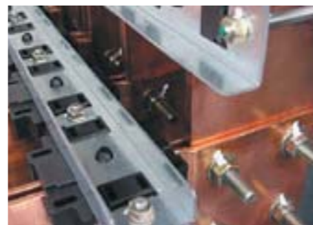
^ Connection on 120 x 10 bars (4000 A)
