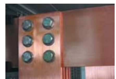
^ Connection on 120 x 10 bars (4000 A)
